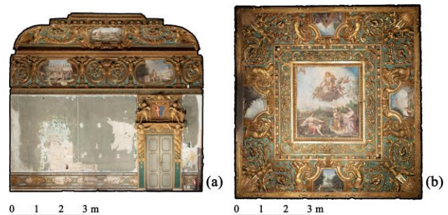
Figure 6. (a) “Green Room” western wall orthoimage (obtained from photogrammetric dataset). (b) Green Room vaulted ceiling orthoimage (obtained from photogrammetric dataset).
