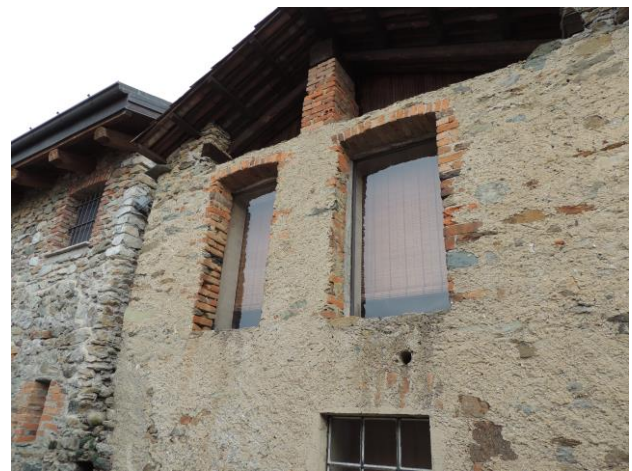
Figure 16. Building F - Intervention preserving both the external masonry surfaces and the roof (credits Silvia Rescic).
