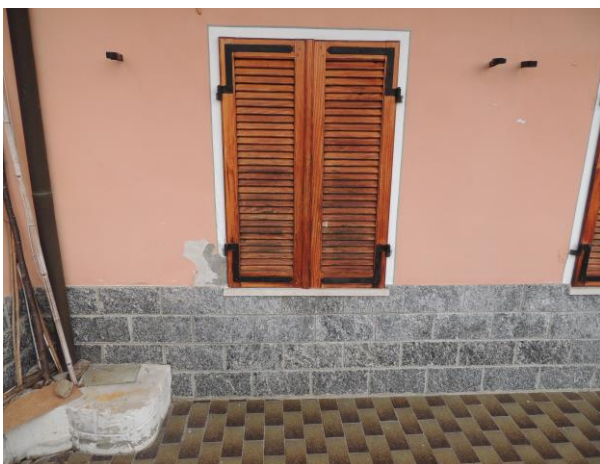
Figure 8. Building E - Baseboard in stone slabs and an external flooring in ceramic tiles, replacement of the windows and application of a new finishing layer (credits Fabio Fratini).
