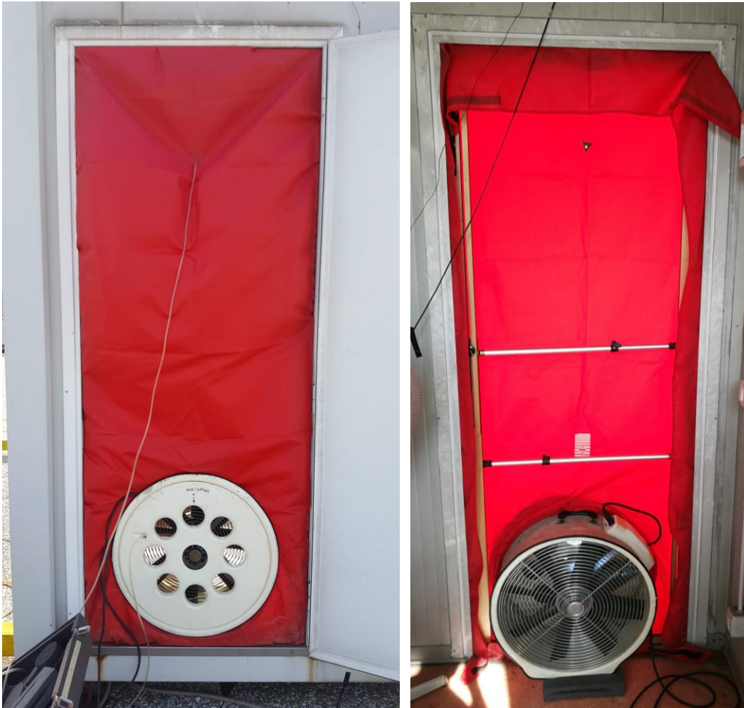
Figure 4.5. Blower door test set-up
