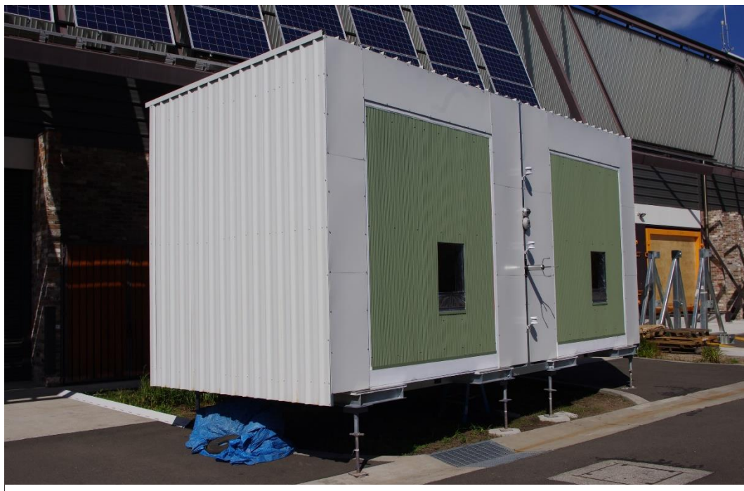
Figure 3.3. Completed test cells
