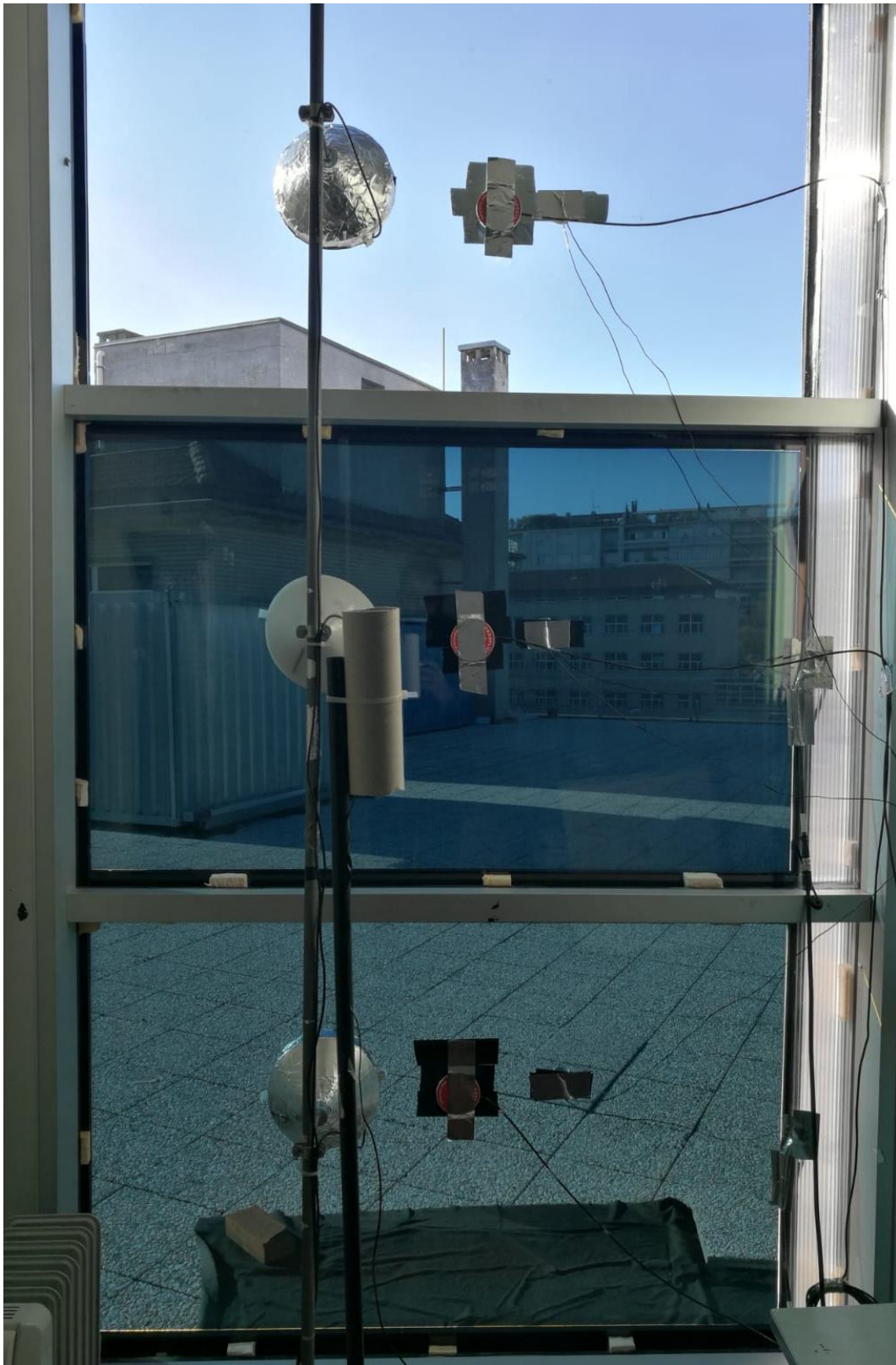
Figure 4.3. Sensors placed on the internal side of the test cell. In each IGU are visible a surface thermocouple (on the right), a heat flux plate (in the centre) and a pyranometer (on the left). In correspondence of the central pyranometer is visible the cardboard cylinder shielding one of the internal air temperature probes.
