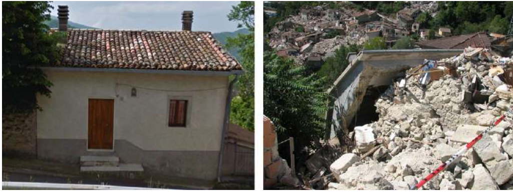
Figure 8. View of the building used as case study before and after the earthquake.
