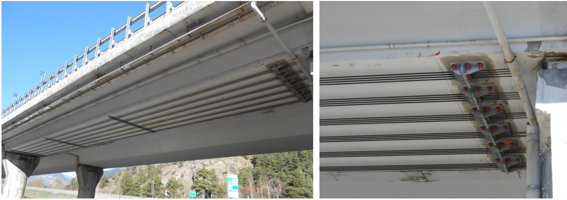
Figure 6.9: External pre-stressing tendons installed for strengthening the structure
