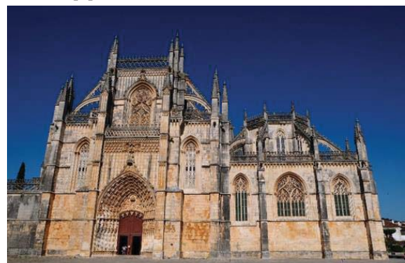
Fig. 1. Monastery of Batalha.
