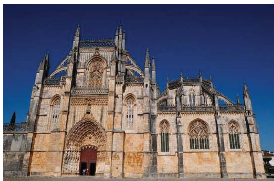
Fig. 1. Monastery of Batalha.
