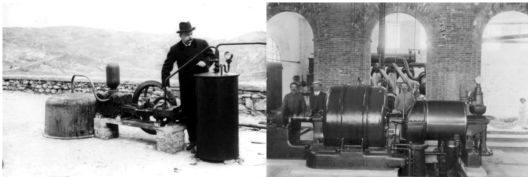
Figure 5.2 left) the experiment of Prince Ginori Conti in 1913: the geothermal energy was converted to switch on five bulb lamps (source https://www.unionegeotermica.it/esperimento_ginori_conti.asp ); right) the first electric power plant “Larderello 1” started operating in 1913 (courtesy of Alessandro Lenzi. Presented during the GEO200 conference in Pisa, May 2018)
