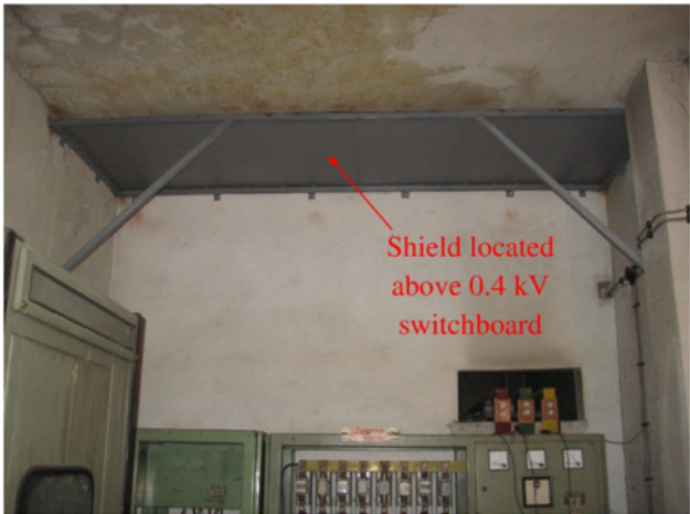
Fig. 6 Shield located above the 0.4 kV switchboard
