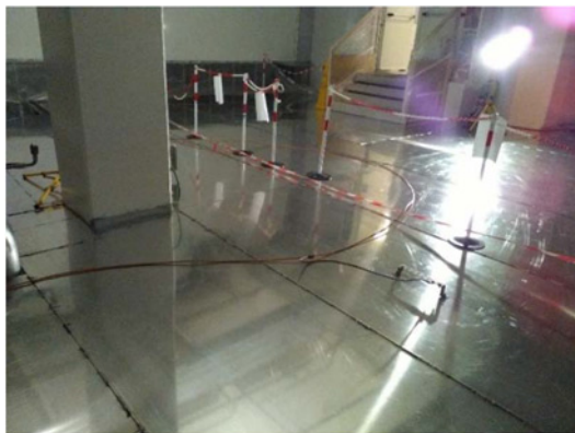
Fig. 13 Picture of the first shield: under the floating floor of the testing area
