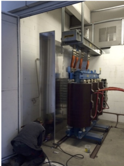
Fig. 1 Local shield for the power transformer
