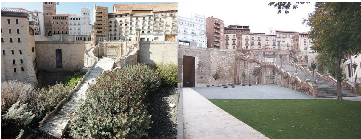
Fig. 7: The monumental stairway of the Paseo del Óvalo built in 1920 in Teruel (Spain).
