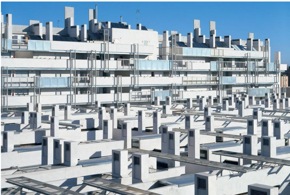
Figure. 1.3. Wind towers in 141 Housing project designed by Morphosis Architects & Begoña Diaz Ugorri Architect in Carabanchel, Spain (Halbe, 2007)
