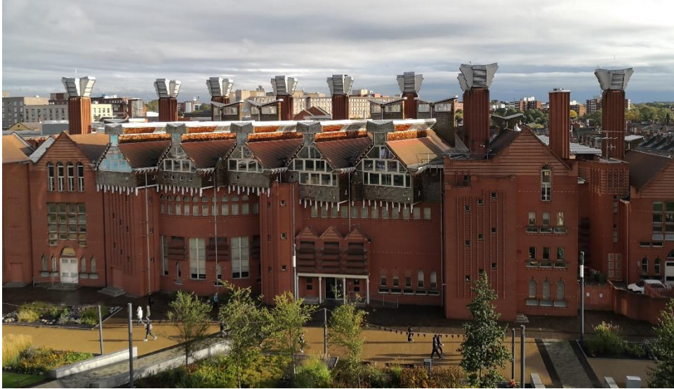
Figure 1.2. Naturally ventilated Queen's Building with its several wind towers at De Montfort University in Leicester, designed by Short and Associates
