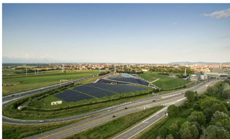
Figure 3. Photo of the Barricalla landfill.
