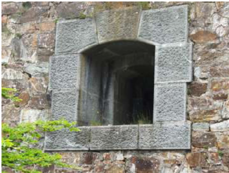
Fig. 6. The frames of the openings (Mattone).
