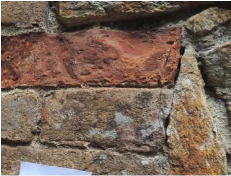
Fig. 15. Bricks of the internal jambs of the tunnel (Fratini).
