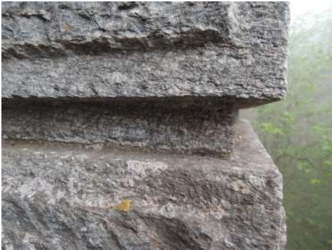
Fig. 8. The angular ashlars (Fratini).
