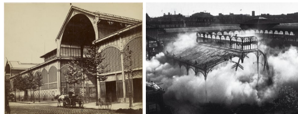
Figure 5. Les Halles of Baltard before and during demolitions in 1971.
