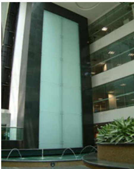
Fig. 33 Water wall for cooling strategy in the atrium of LEO Building in Putrajaya, Malaysia.
