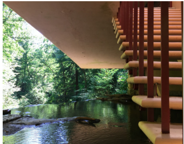
Fig. 7 Bear Run: the staircase to the water.
