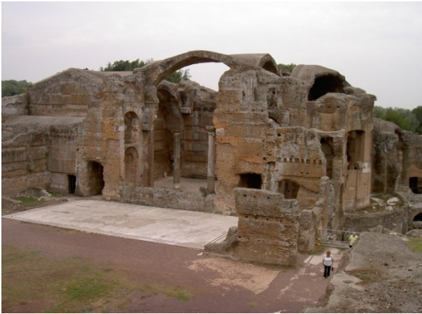
Fig. 1 The thermae complex in Villa Adriana, Tivoli, Italy.
