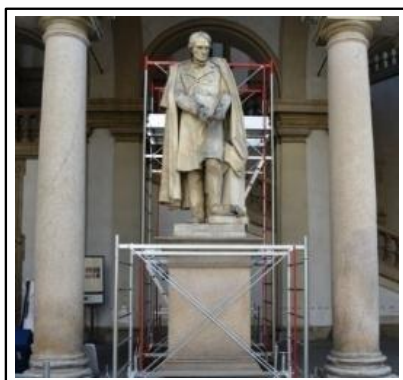
Fig. 2: Initial phases of the conservation of Antonio Galli's sculpture of Carlo Ottavio Castiglione (1855). Height of statue plus the pedestal 503 cm (198 inches), Just the statue 305 cm (120 inches). The original surface appears hidden by a layer of aged protective varnish.
