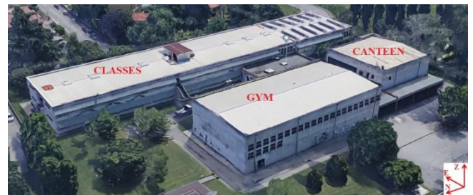
Figure 3. Building overall view
