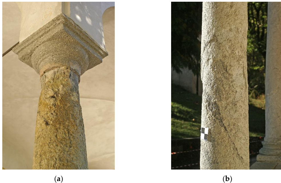
Figure 7. Different types of surface material degradation on the columns of the Via Crucis portico: (a) erosion; (b) exfoliation.
