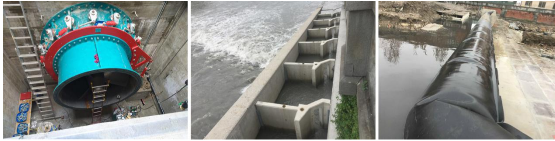
Fig. 10. The first picture show the positioning of Kaplan Turbine, the second one shows vertical slots of fish pass and the third one shows the inflatable check dam (Authors, 2017).
