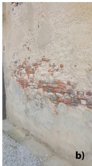
Fig. 1. Some examples of plaster detachment on historical walls due to: a) damp action from capillary rising, b) the action of freezing-thawing cycles.
