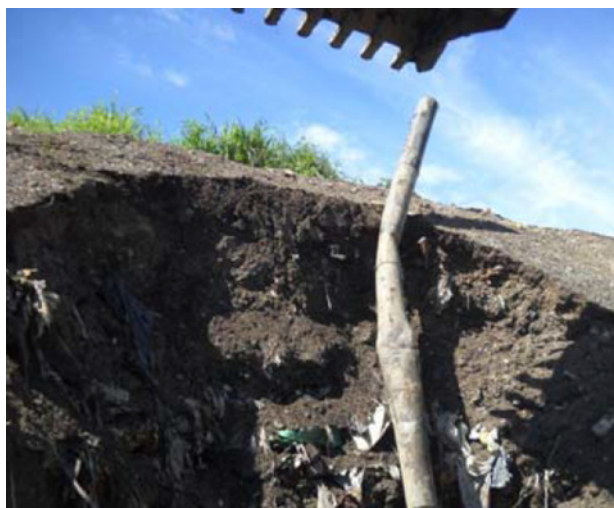
Fig. 4. Temporary covering of non hazardous waste dump with engineered material arising from mixed soils, glass, debris from clean water sedimentation (credits Oggeri 2014).
