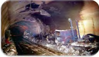
Ruins of the Mont-Blanc tunnel fire (1999) Fire duration: 53h; Fatalities: 39 (including a firefighter and a security guard).
