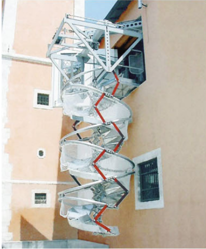
Fig. 5 | Legislative requirements for safety in historic buildings: helioid retractable staircase (credit: design by Nucleo, Vegaprogetti and Cip – TO; production by Borini Engineering, 2003).
