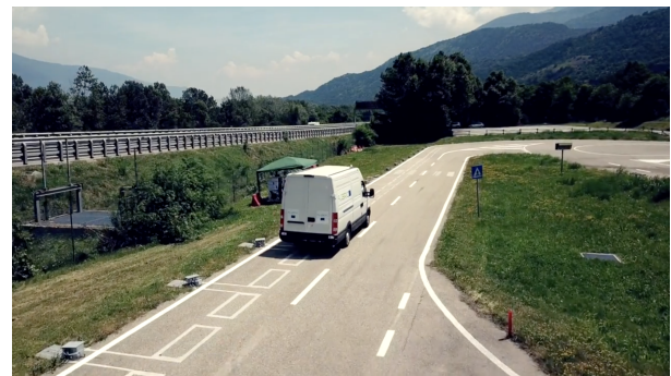
Fig. 16: The EV in the charging lane.
