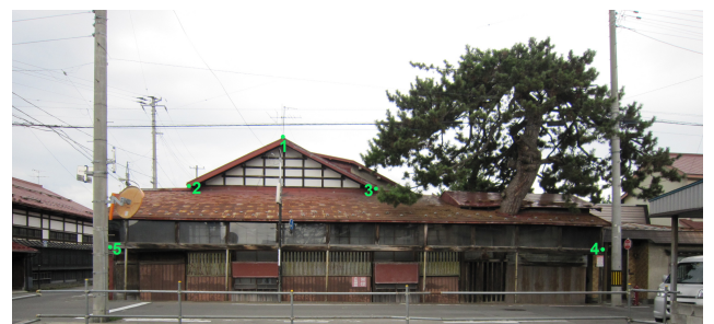
Figure 8. Feature points manually chosen for the Former Matsuno-Yu building.
