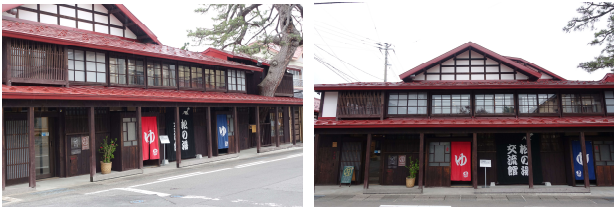
Figure 4. Pictures of the Former Matsuno-Yu building from on-site survey in 2018 after the restoration.
