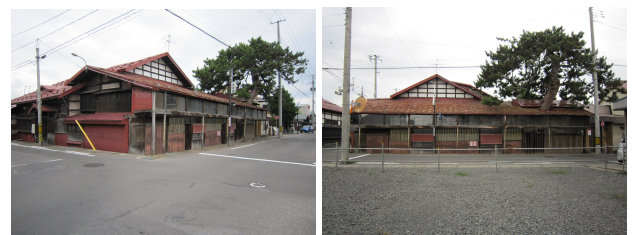
Figure 3. Pictures of the Former Matsuno-Yu building from local archive before the restoration in 2013.
