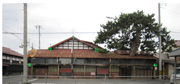
Figure 8. Feature points manually chosen for the Former Matsuno-Yu building.
