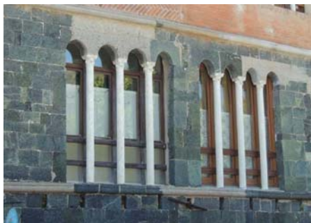
Fig. 03 : Serpentinite in regular blocks (on the left) and in column and capital (on the right)
