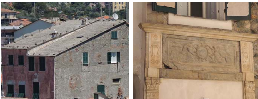
Fig.05 : Slate as roof tiled (on the left) and in a bas-relief (on the right)
