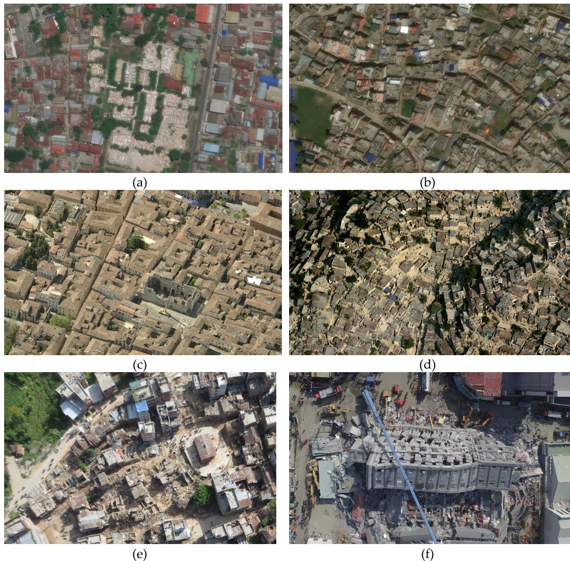
Figure 1. Examples of building damages caused by earthquakes captured in satellite (first row), airborne (second row) and UAV (third row) images, respectively. In detail: (a) Indonesia, 2016; (b) Nepal, 2015; (c) Italy, 2009; (d) Haiti, 2010; (e) Nepal, 2015; (f) Taiwan, 2016. The damage looks different depending on the considered spatial resolution, off-nadir angle and building typology.
