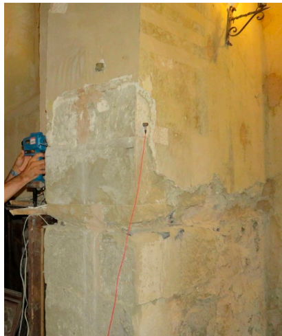
Figure 7. Impact test on single big sandstone constituting the masonry texture.
