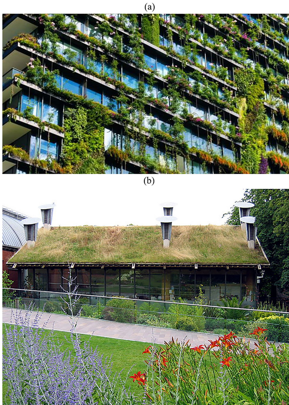
Fig. 6. Examples of (a) green wall in Sydney (Courtesy: dr. Irene Soligno) and (b) aesthetic green roof at the Horniman Museum in London, UK (Reproduced without modifications under Creative Commons license CC BY-SA 2.0; author: secretlondon123).
