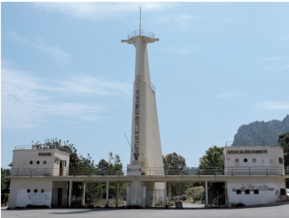
FIG. 2 Palermo, ex Istituto "F. D. Roosevelt": edificio di ingresso Palermo, former "Institute F. D. Roosevelt": entrance building
