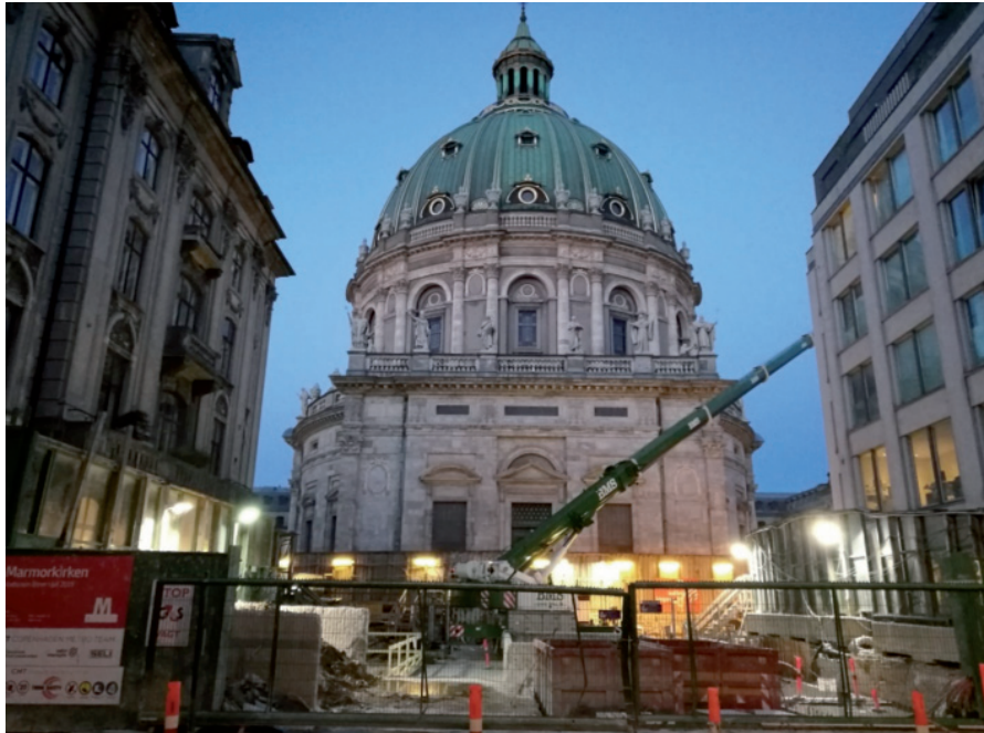
FIG. 1 Copenhagen, Danimarca, progetto Cityringen Metro Copenhagen, Denmark, Cityringen Metro Project
