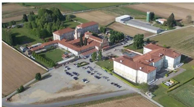
Figure 1. The whole complex with the health care building on the right and the Church and cloister on the left.
