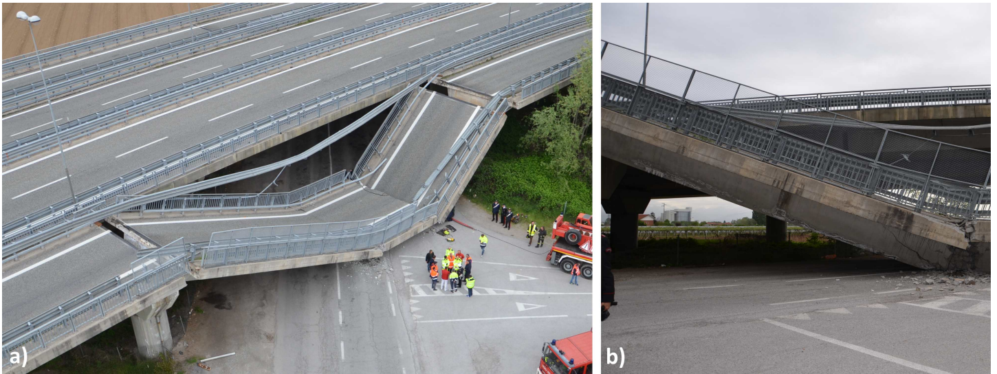
Figure 1: a) collapsed structure. b) in-situ casted intact joint.
