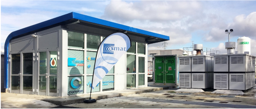
Fig. 12 – DEMOSOFC plant with 2 SOFC modules in operation (December 2018). On the left, the technical building where the control room and the electrical cabinet room are located. In the central part, the first SOFC module. On the right, part of the biogas cleaning and compression container.
