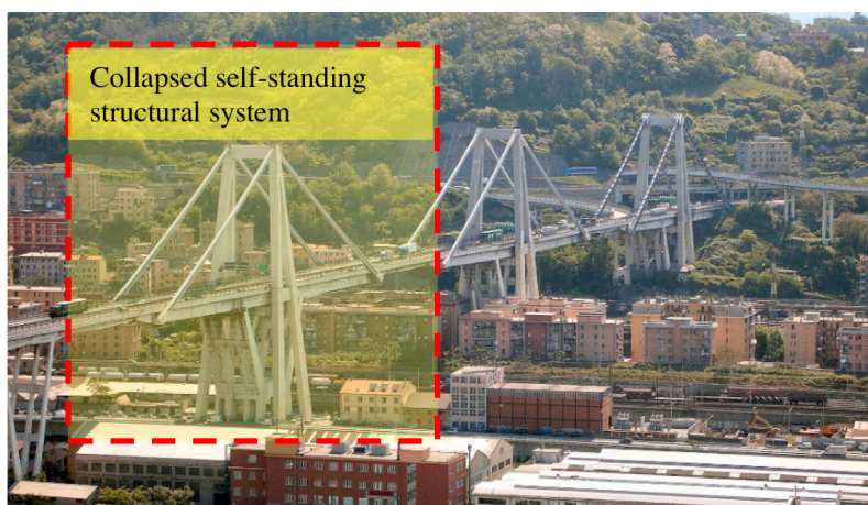
Fig. 1. Three self-standing structural systems of Polcevera Bridge.
