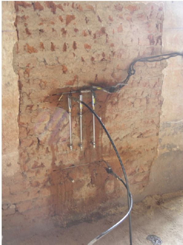
Figure 4: Flat jacks test carried out at the Royal Palace of Venaria.
