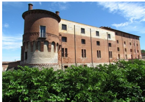
Fig. 1- Saluzzo Castle, view overlooking the hillside
