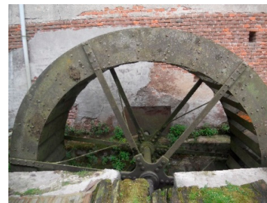
Figure 5. The overshoot water wheels of the Riviera mill: (a) Before the renovation (Courtesy of Arch. Roberto Olivero, 2004); (b) after the renovation.
