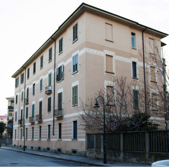
Fig. 3. The 1920s test building in Torino.
