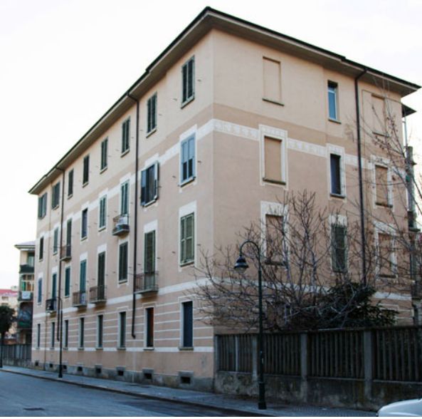
Fig. 3. The 1920s test building in Torino.
