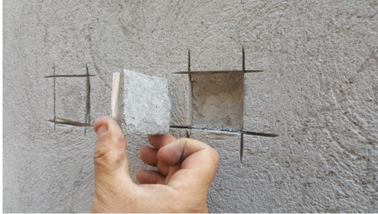
Figure 133: Test area to be patched back.
