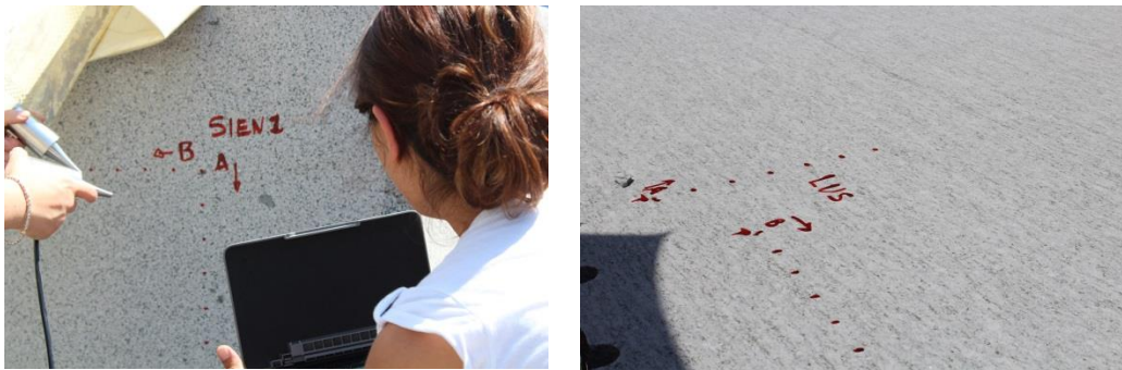
Figure 30: Ultrasound Pulse Velocity measurements in situ on blocks.
