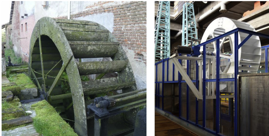
Fig. 10. Breastshot water wheel in Verolengo, Italy and its laboratory 1:2 model [201]. Source: authors' compilation.
