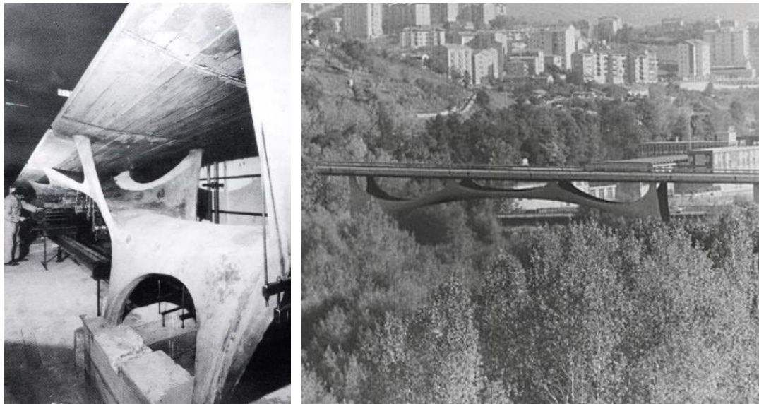
(a) (b) Figure 3: Bridge on Basento, Potenza, Italy, (Iori & Poretti, 2007): (a) model in laboratory; and (b) real structure.
