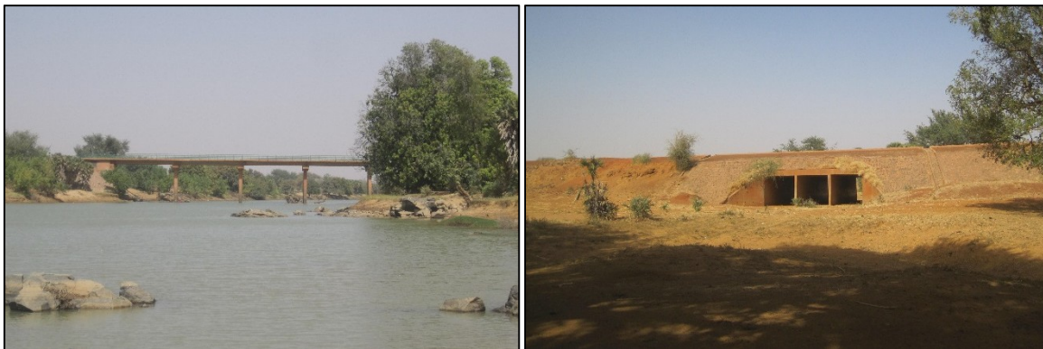
Figure 5. Left: The Farié bridge on the Sirba River. Right: the culvert with three opening placed on the left overbank.
