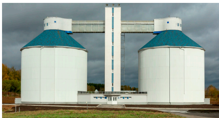
Figure 2. Digesters at northern wastewater treatment plant (WWTP) in Ekaterinburg, Russia.
