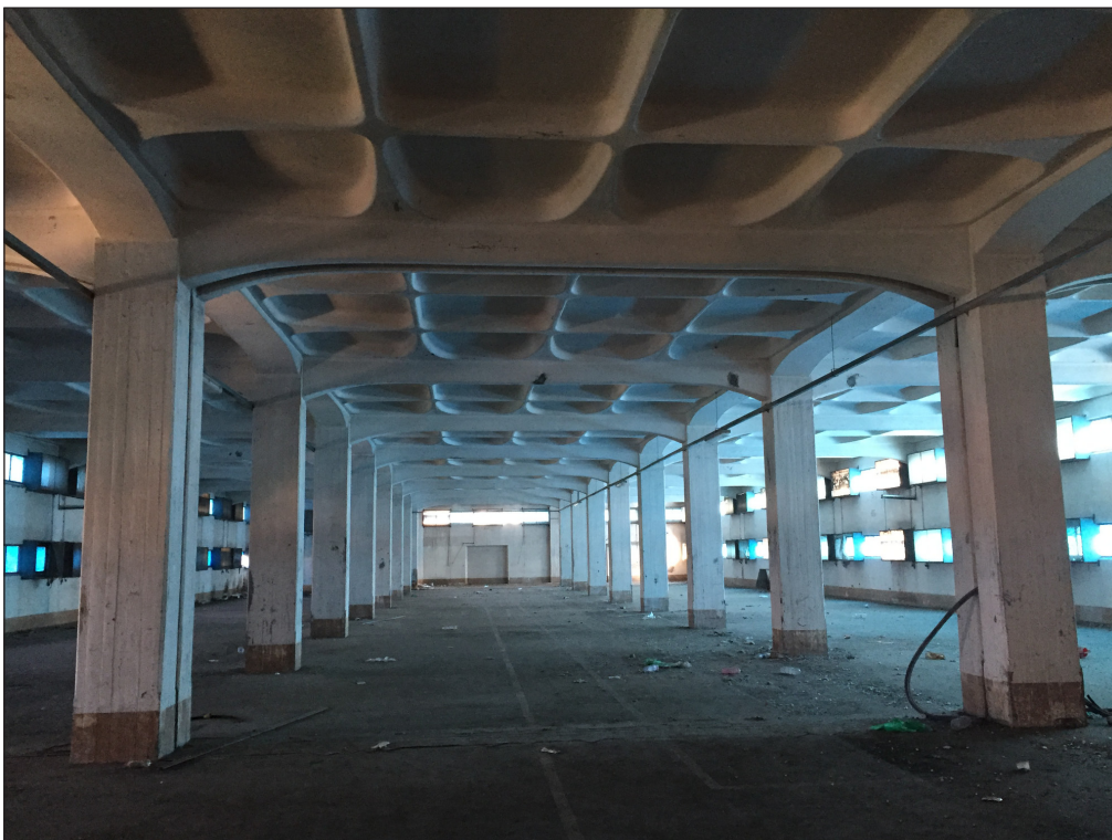
Figure 6: Concrete slabs of the 'Ballette' Building, Manifattura Tabacchi, Bologna. Photo by Micaela Antonucci, 2017.
