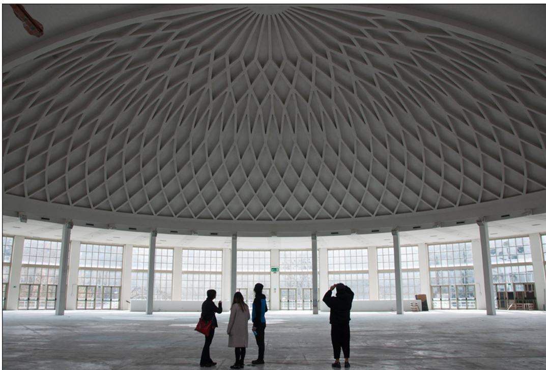
Figure 4: Pier Luigi Nervi, Hall B of the Torino Esposizioni in Turin, 1947–54. Photo by Sofia Nannini, 2018.
