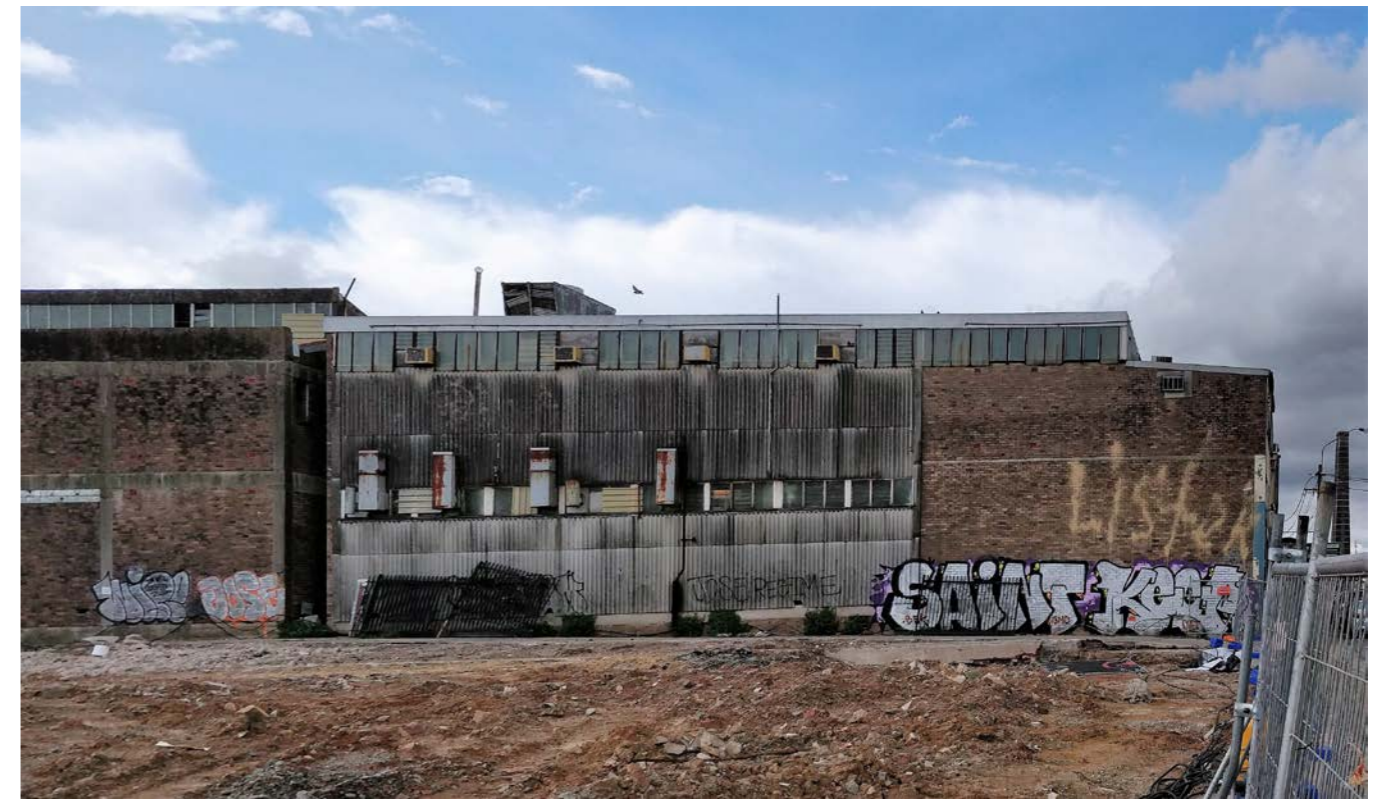
Image 6. Undergoing demolition of the warehouses surrounding Tortuga Studios, in St Peters.
